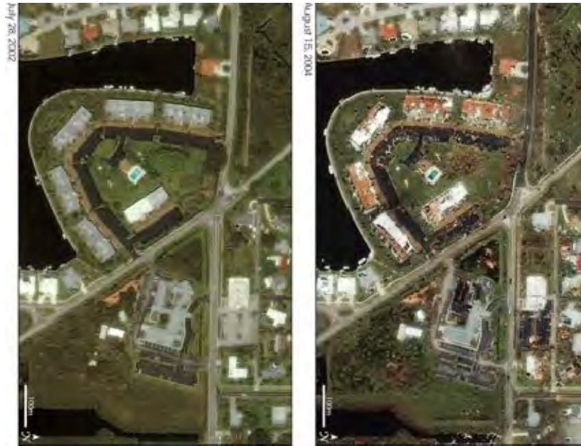
Figure 9. Low resolution pre (left) and post-storm (right) satellite imagery showing damage to buildings near inland water bodies with scattered debris. (NASA Earth Observatory, 2004)
